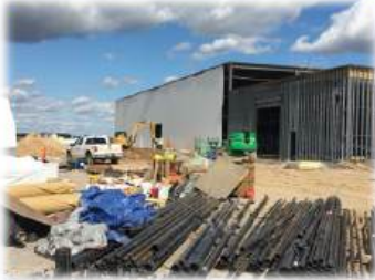
Construction of 135k sq. ft. Pinconning cultivation facility commences
